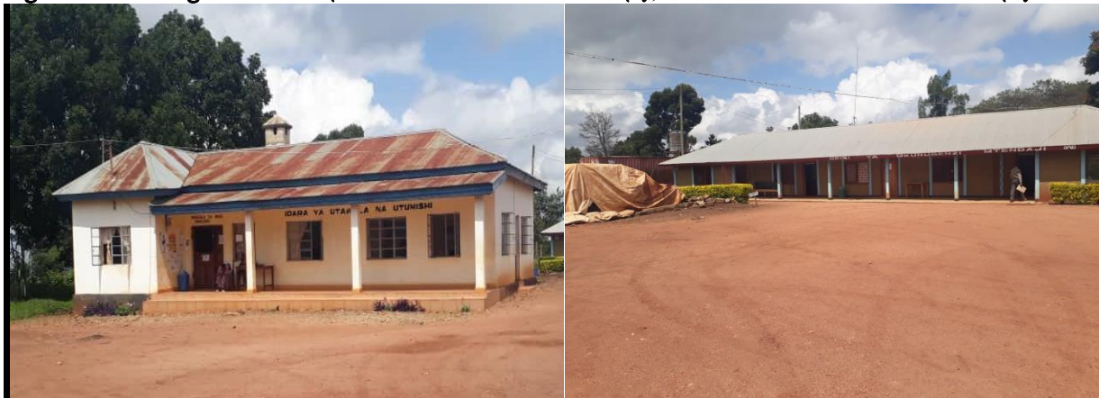
Figure 3: Existing Structures (Internal Auditor's Office (L), Generator and Store Rooms (R))
