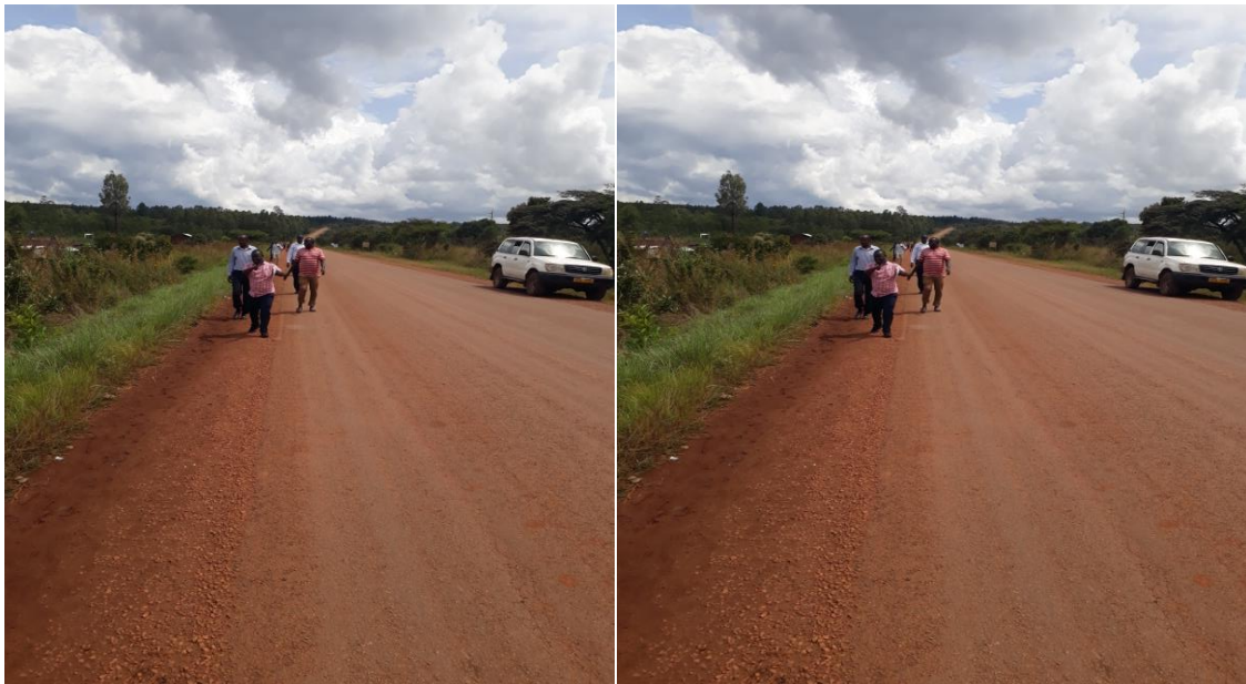
Figure 3: Access Road to Project site
